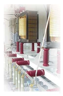
Above two pictures shows how NEPSI interconnects components with Silver or Tin-plated Copper Bus Bar. This method of interconnection is not prone to failures associated with forces during capacitor bank energization. Over the life of the equipment, air provides the best insulation medium as it does not allow for tracking or treeing that is common with solid dielectric cables. See the following link for further information on Phase and Ground Bus System.
